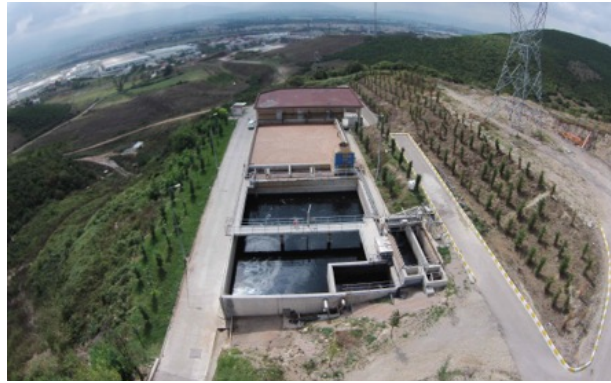
Pic.9: IZAYDAŞ Wastewater Treatment Plant
